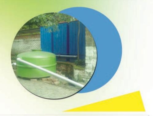
io-Digester is a decomposition mechanized toilet system which decomposes Human Excretory Waste in the digester tank using specific high graded bacteria further converting it into methane and water, discharged further to the desired surface.
